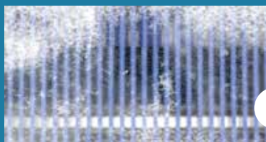
outdoor unit frosting
